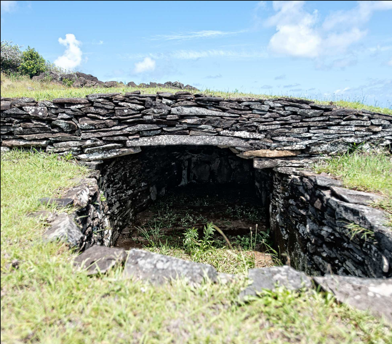
Partially restored, Orongo stone house.
